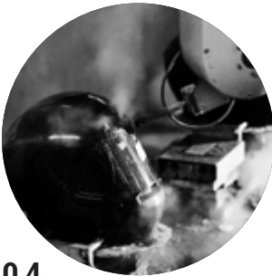
04 Openings are cut with high-pressure waterjet technology.
